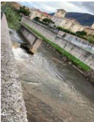
Figure 1. the Alveo Comune Nocerino river culverted in Domenico Rea street
