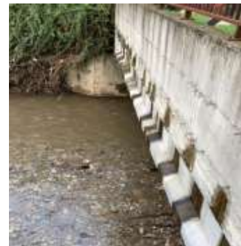
Figure 2. the Alveo Comune Nocerino river culverted in Domenico Rea street
